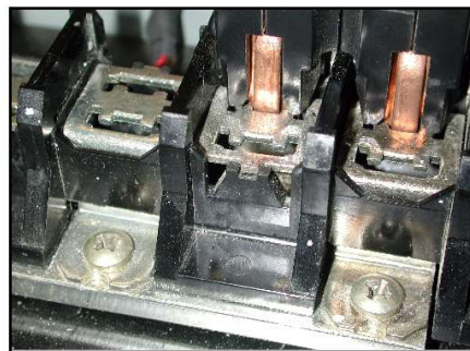
B. "Z" clip, clamped to bussbar with 10-32 screw.
